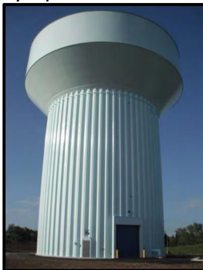
Source: Rochester Public Utilities
