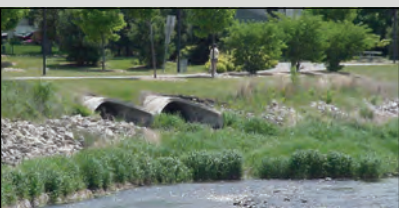
Storm Water Management
