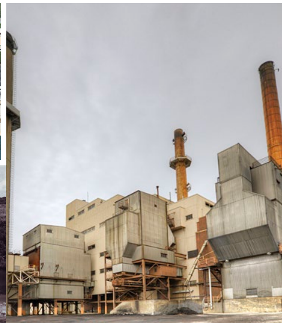
Coal yard scrapped clean of all coal. Taken at the end of November 2013.
